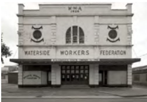
Waterside Workers Hall, 2019, Tony Kearney
