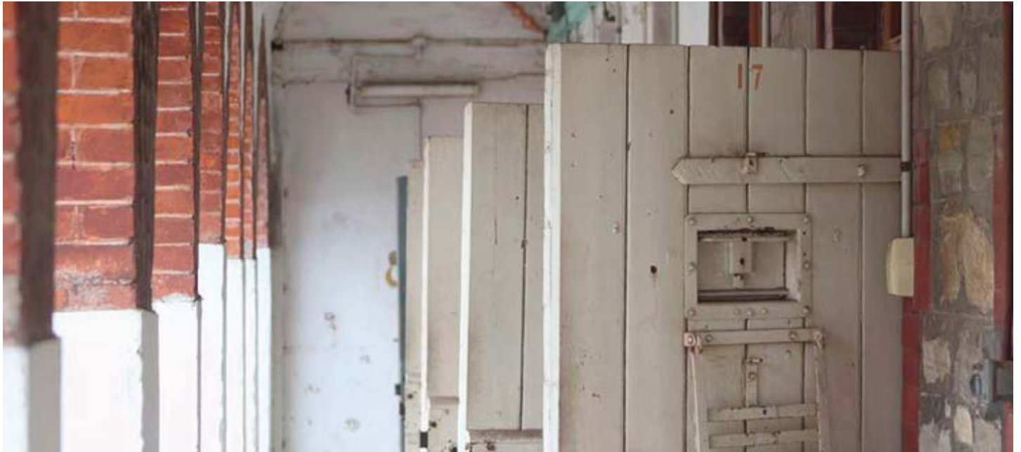
Adelaide Gaol, Cell Doors, Yard 4, image courtesy Adelaide Gaol
